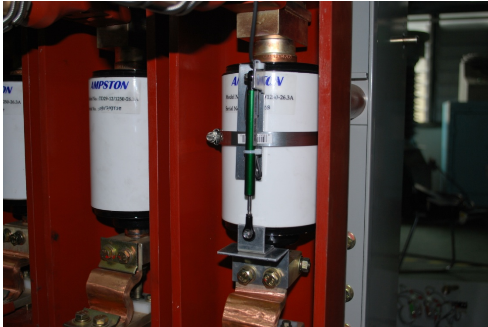
Resistor Transducer on Vacuum Circuit Breaker
